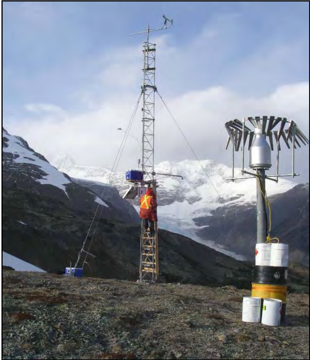
Figure 18.24 Met Station Installation Near the Brucejack Lake Camp.
