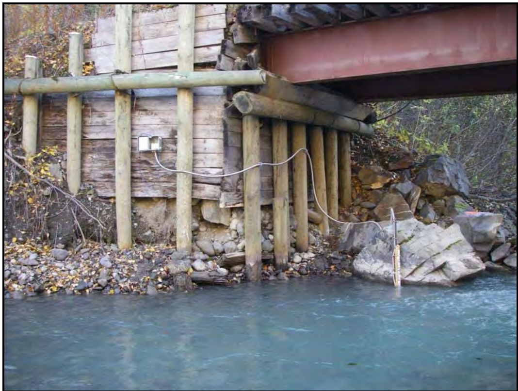
Figure 18.25 Hydrological Station on Scott Creek
